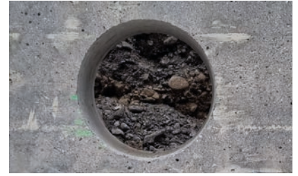
1. Carottage \varnothing 250 mm
