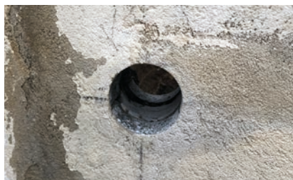
Carottage \varnothing 70 mm
