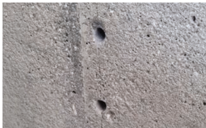
2. Fori praticati \varnothing 12 mm
