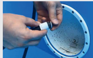
Threading in the cable gland
