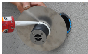
3. Mount the base element, apply additional adhesive if necessary
