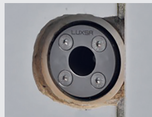
Nozzle base element mounted in defective thread
