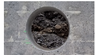
1. Core drill hole \varnothing 250 mm
