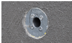
5. Base element sealed with liquid liner
