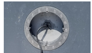
5. Cable pulled in and sealed with Press & Close system
