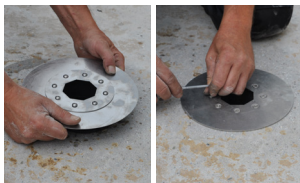
5. Set base element and tighten with spanner
