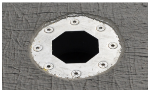
6. Base elements sealed with liquid liner
