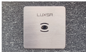
6. Finished tiled pool with Q-Line nozzle cover
