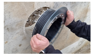
3. Insert base element into drill hole
