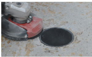
3. Grinding a slight gradient
