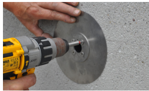
4. Tighten the base element
