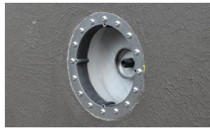
4. Sealed with liquid liner
