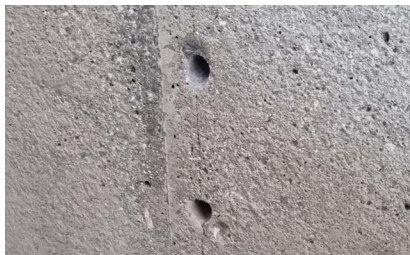
2. Fori praticati \varnothing 12 mm
