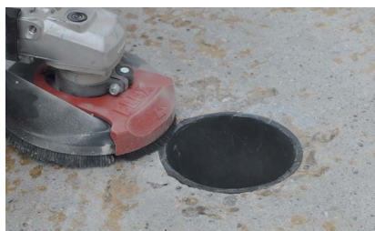
3. Grinding a slight gradient
