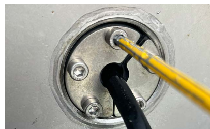
3. Tighten the Press & Close cable seal by hand or with a cordless screwdriver
