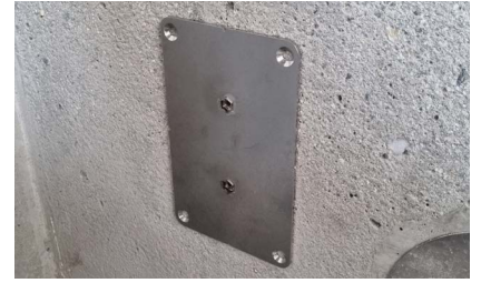
3. Mounting flange can be set, holes drilled for fastening
