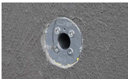
5. Base element sealed with liquid liner
