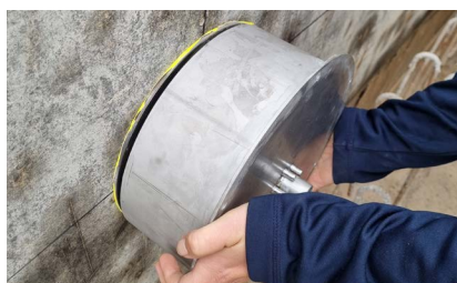
3. Tighten the installation housing as far as it will go
