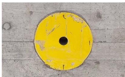
4. Installation housing with formwork protector set in concrete
