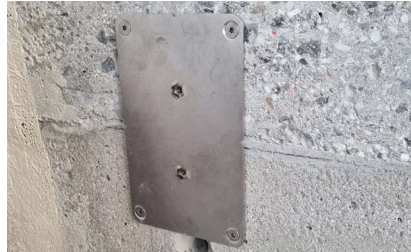
5. Fully assembled mounting flange
