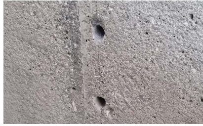
2. Drilled holes \varnothing 12 mm
