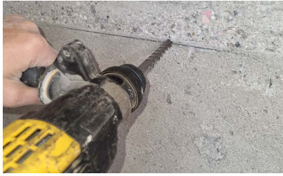
1. Drill hole for the threaded sleeve of the mounting flange
