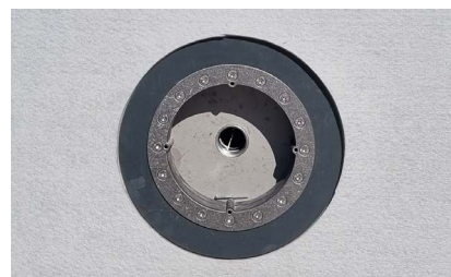
4. Base element set and ready for film installation
