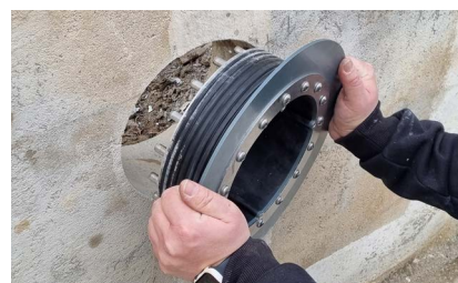
3. Insert base element into drill hole
