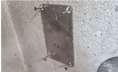
4. Mount the mounting flange with screws and dowels
