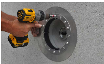
3. Tighten the base unit, do not install until walls have been re-profiled
