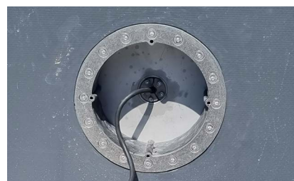
5. Cable pulled in and sealed with Press & Close system
