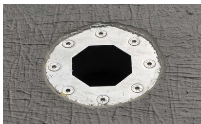
6. floor drain sealed with liquid liner
