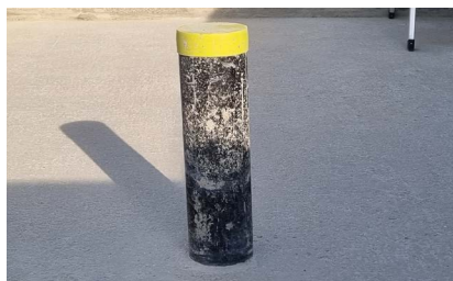
1. PE pipe inserted in base plate
