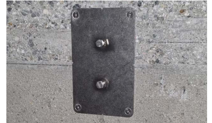
6. Screw in the screw to protect the blind holes
