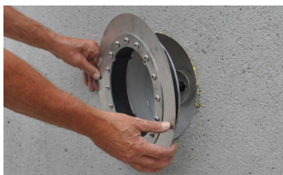
2. Place and align the base element
