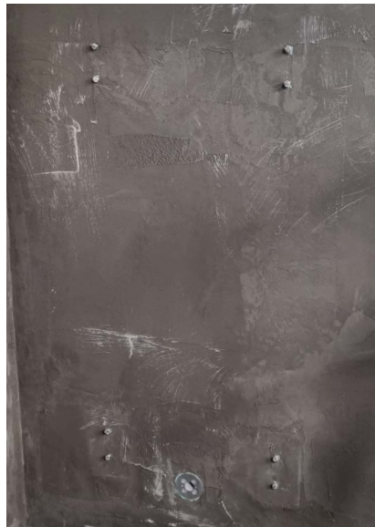
8. Waterproofing has been applied
