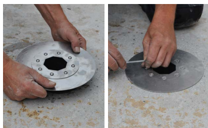
5. Set base element and tighten with spanner
