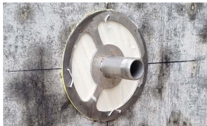
1. Nail the formwork protector to the formwork
