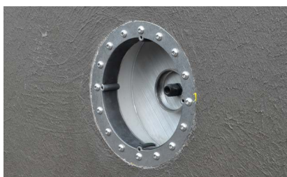
4. Sealed with liquid liner
