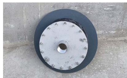
2. Base element refurbishment
